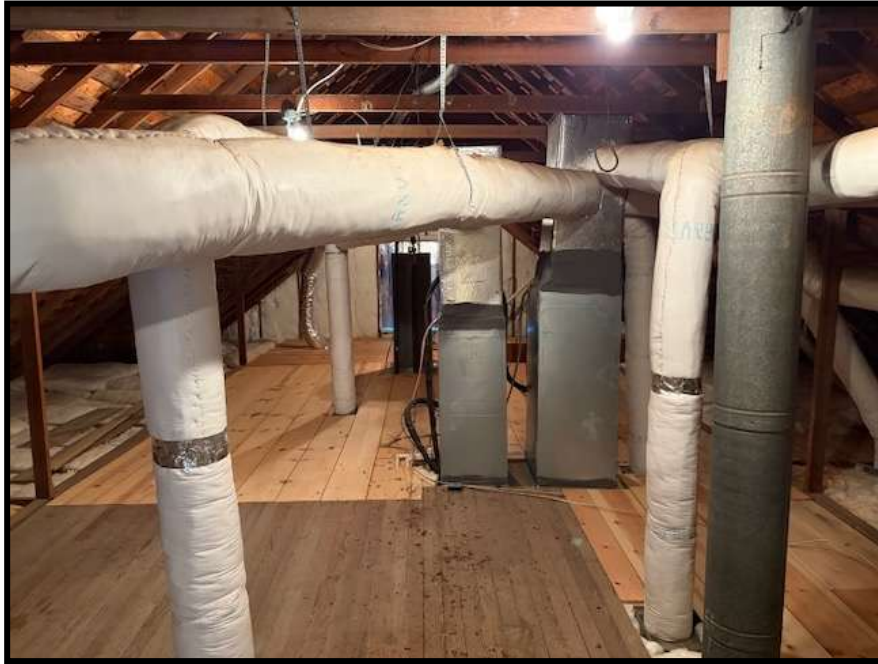
13. Attic Used For Storage And HVAC.
