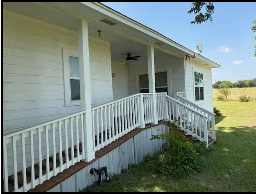
9. Back Porch On South Side Of Residence.
