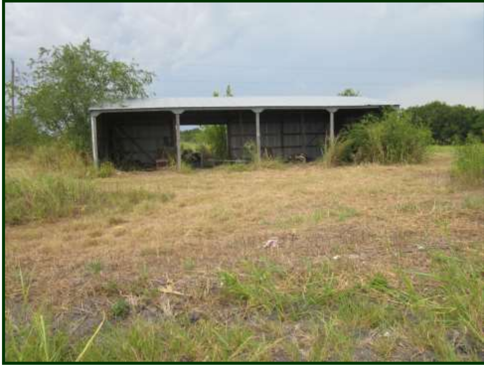
Metal Building Near Old Homesite. Jonah Water Meter And Electric Meter On Site.
